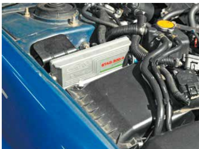
Fig. 6 Recommended position of the installed autogas controller
